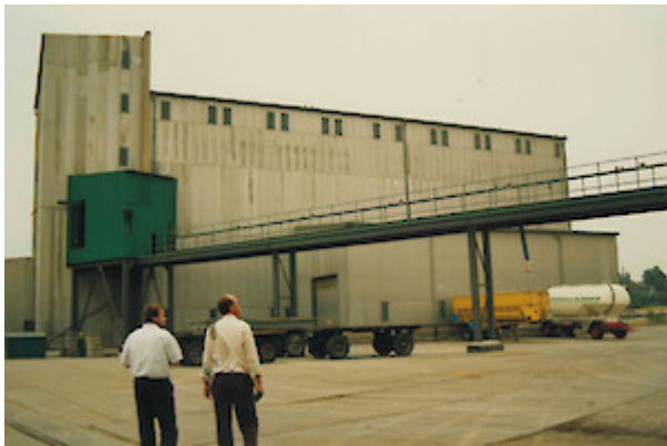
Main building of the plant with neighbouring loading ramp (© Deutsche Tiernahrung Cremer)
