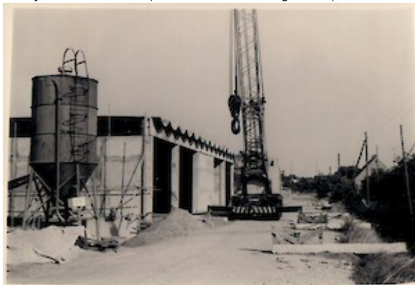
A photo from the construction phase: A crane stands next to shell structures (© Deutsche Tiernahrung Cremer)
