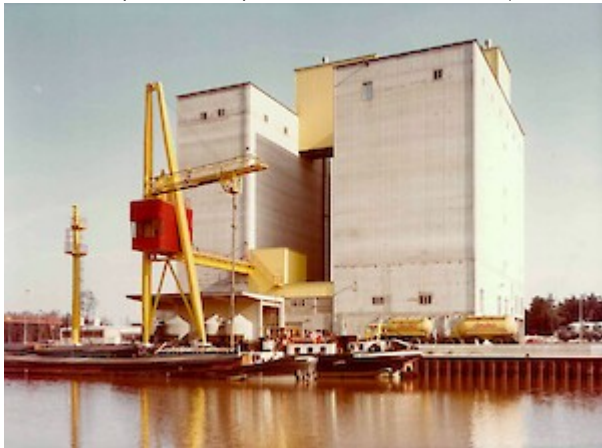
The pig feed plant in Bramsche shortly after its completion (© Deutsche Tiernahrung Cremer).
